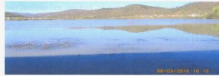
Pic. 2.5. The silted area of the Rioni HPP dam reservoir
